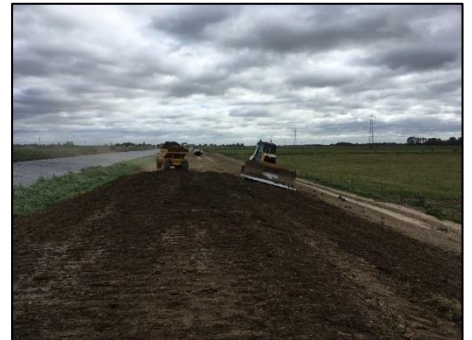
Strengthening works of Cradge Bank
