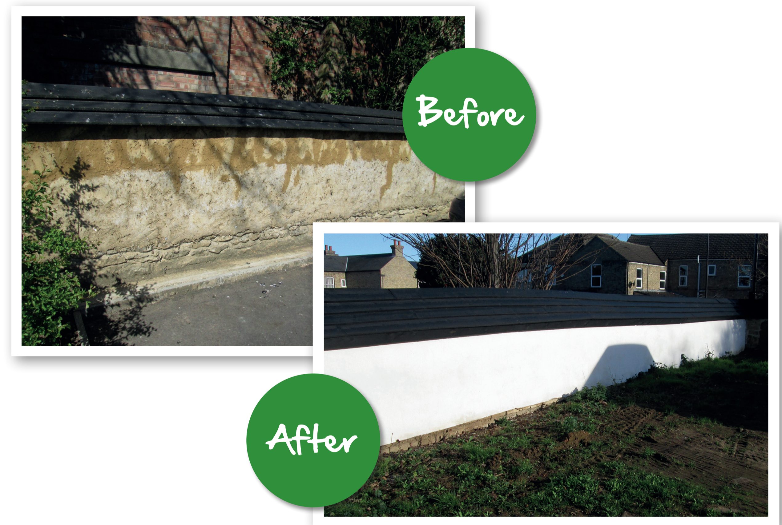
The mudwall at the Black Bull Public House on Market Street before and after it was restored in 2017.
