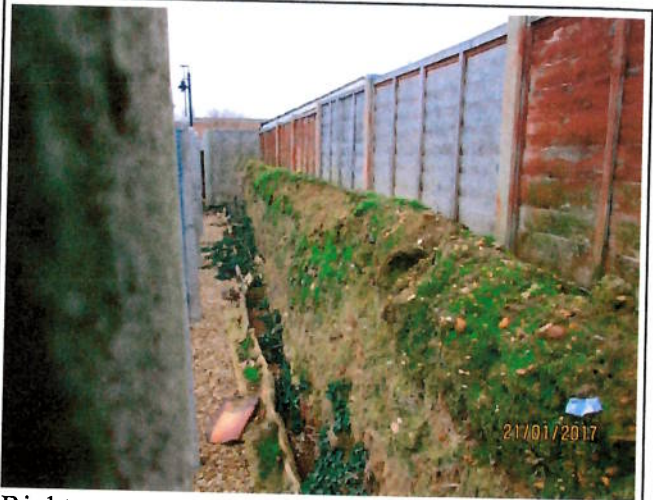
Right R/H end of wall
