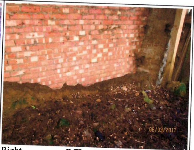
Right R/H end of wall
